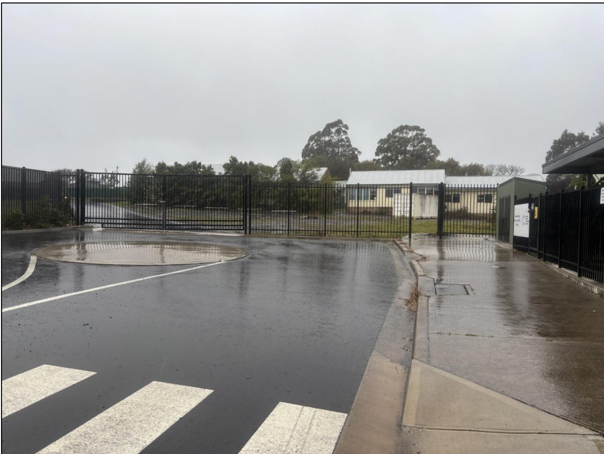
Figure 4: Internal site entry looking towards the south from the internal driveway.
